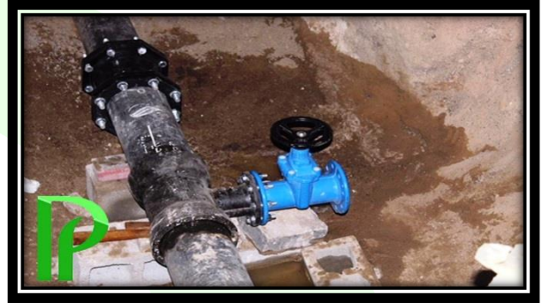
Bawadi Mall - D.I Main Line Modification Works
