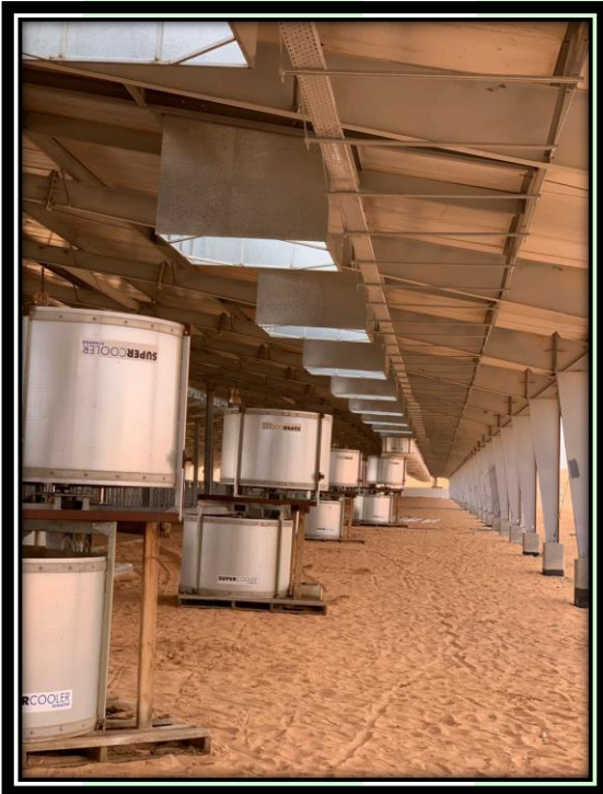
Al-Ain Farms for Livestock Production - Installation of Korrakool Fans
